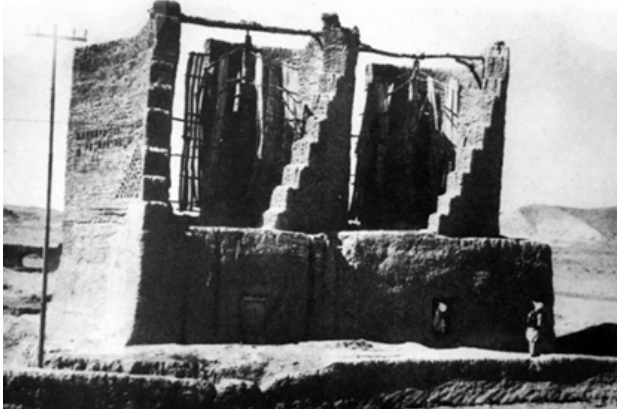
Fig. 6. The photo of a windmill in Sistan. Photo: Richard Hewer, 1971; Source: Beazley, Harverson & Roaf, 2013.
