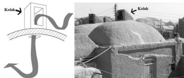
Fig. 1. A kolak in Qaleh-no Village (right); A graphic representation of how the wind enters the room (left). Source: Heidari, 2015.
