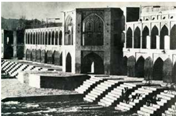
Fig 2. Khaju Bridge. Source: Blunt, 1966.
