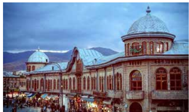
Fig. 7. Baroque-style buildings in Hamedān Imam Square. Photo: Farshad Bahrami, 2016.
