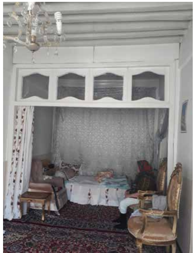
Fig. 5. Two wooden separators in houses 2 and 4. Source: authors' archive.
