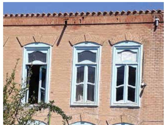
Fig. 7. Brickwork on the facade of the house No. 9. Source: authors' archive.
