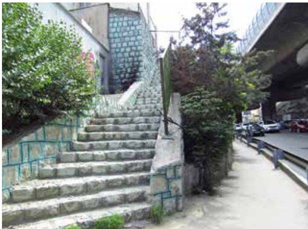
Fig. 7. The non-inclusive stair structure of the sidewalk neglecting the rights of disabled people. Source: authors' archive.
