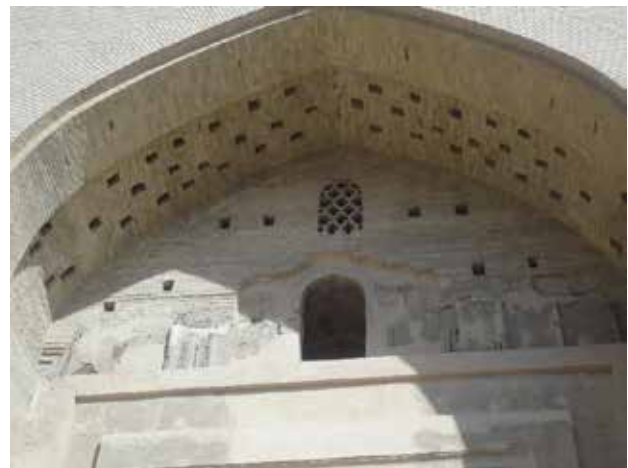
Fig 4. Gypsum coating below the Haroonia entrance door. Photo: Hossein Kouhestani.2017.
