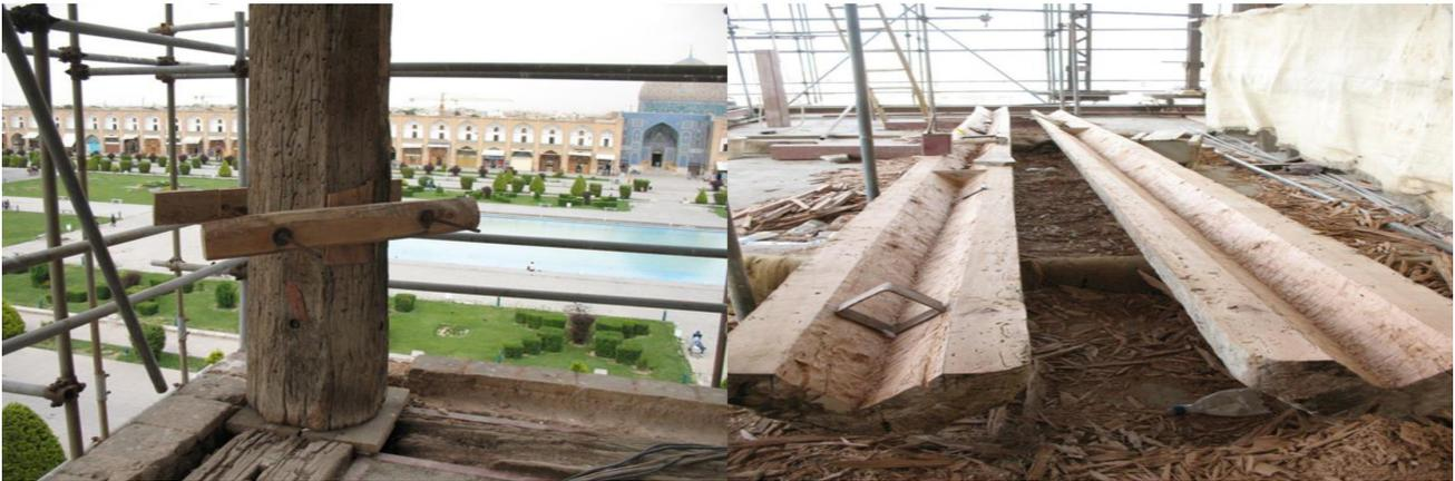
Fig. 2. Latent intervention in in restoration of columns in Ali Qapu. Photo: Reza Abouei.
