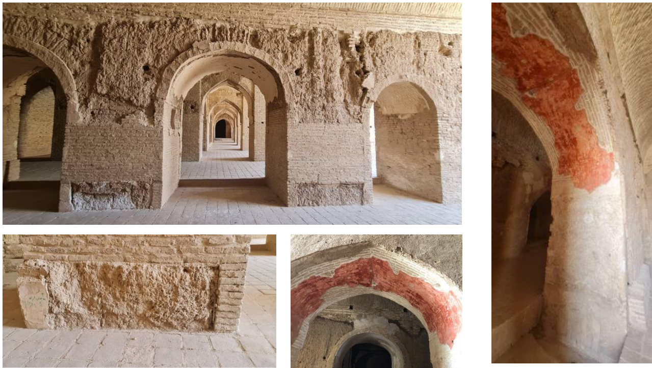
Fig. 2. Shabestan and eastern porch, a brick wall covered with red plaster. Photo: Seyed Amir Mansouri, 2022.
