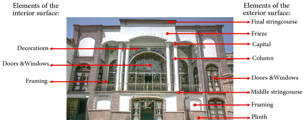
Fig. 3. Facade elements of Kuzehkonani historical house with the execution method of combined semi-open space in the pattern of a columnar porch. Source: Authors.
