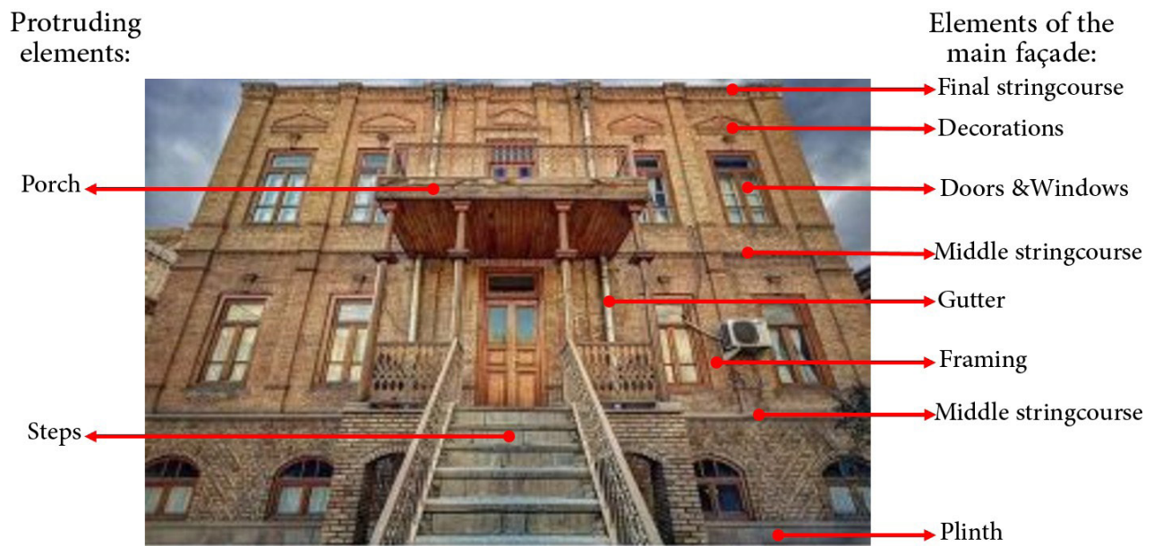
Fig. 6. Elements of the facade of the Siqat-al-Islam historical house in two main and protruding surfaces in the flat facade pattern. Source: Authors.
