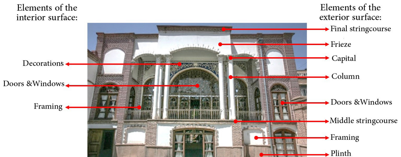
Fig. 4. Facade elements of Heydarzadeh historical house with the execution method of the top semi-open space in the pattern of a columnar porch. Source: Authors.
