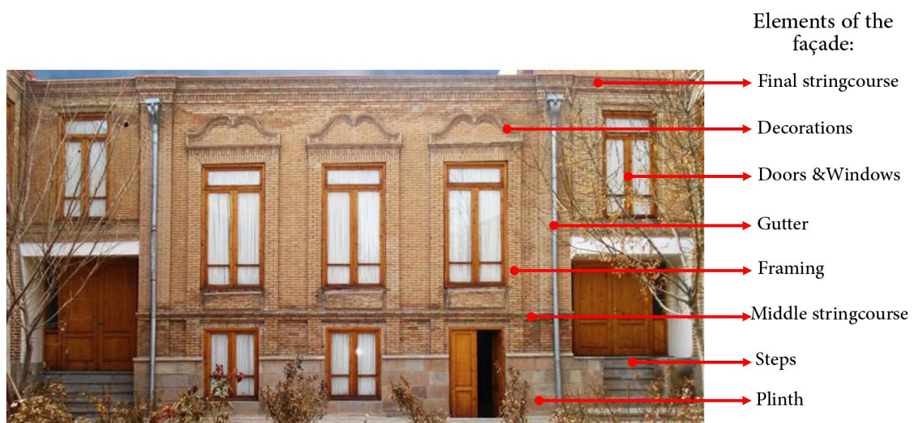
Fig. 5. Elements of the façade of the Solhjoo historical house on the main surface in a flat facade pattern. Source: Authors.
