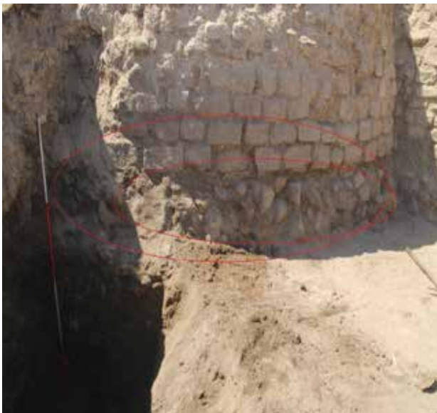
Fig. 12. Eastern walls of castle indicating two types of architecture, one with uncut pebbles and second with cut or so-called Malone stone. According archaeological expedition of Ujan the first dates to Seljuqs reign, whereas the second is from Ilkhanid period. Source: Velayati, 2019.
