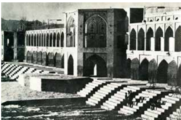
Fig 2. Khaju Bridge. Source: Blunt, 1966.
