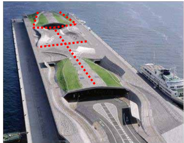
Fig. 8. A view of the complex roof and the directions of movement. Source: https://www.farshidmoussavi.com/node/15#yokohama_international_port_terminal_yokohama_japan_15_54
