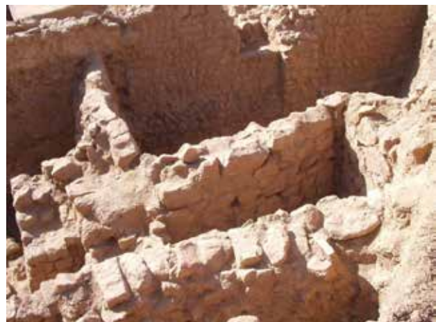
Fig. 3. The plain walls with no lime working traces in the architectural structure of the Rab'e Rashidi, so-called as the Ilkhanate bath. Source: After the authors.
