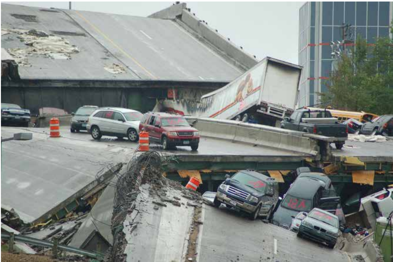
Fig. 3. Minnesota- USA- 2007: the collapse of I-35W Mississippi River Bridge became a symbol of the debilitated state of the once- noble Interstate Highway System- and of what any critics see as America’s disinvestment in its infrastructure. Source: Brown, 2014: 2.
