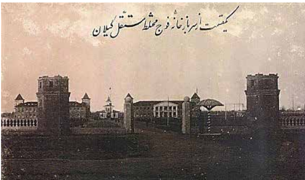
Fig. 3. Gilan Barracks. Source: Archives of the Gilan Cultural Heritage Bureau.
