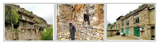
Fig. 4. Stone, wood and soil are the main materials of construction on Hawraman. Source: authors.
