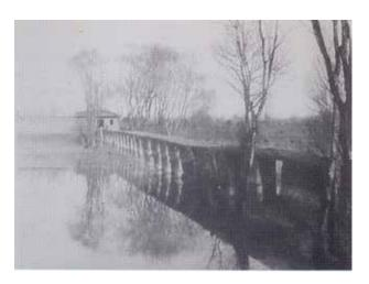
Fig. 5. Wooden bridge of Bahrol-eram in 1891; composed of 29 stone pillars and a wooden floor, which provided the only access to the lake, located along the street leading to Sabze Meidan. Source: Elahi, 2006: 19.
