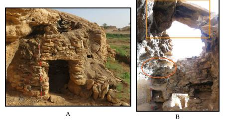
Fig. 4. a. Southern view of space b) entrance to the space. Source: authors. b) Internal view of space b) Arched and combined roof. Source: authors.
