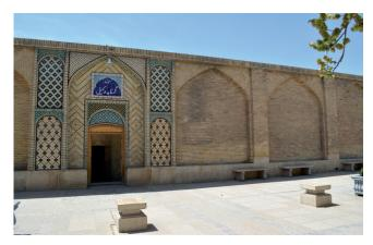
Fig. 1.a. Brick framing in the exterior façade of Zandiyeh buildings.
