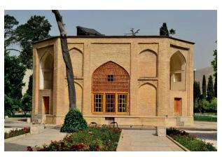
Fig. 1.b. Brick framing in the exterior façade of Zandiyeh buildings.
