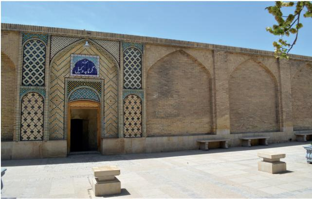
Fig. 1.a. Brick framing in the exterior façade of Zandiyeh buildings.
