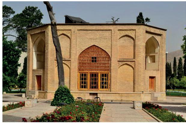
Fig. 1.b. Brick framing in the exterior façade of Zandiyeh buildings.
